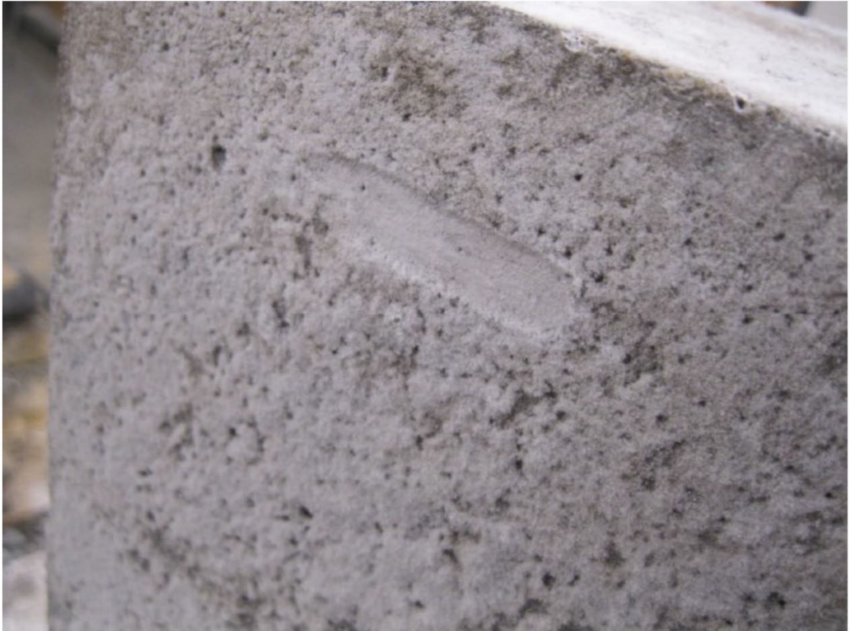
Laboratory photograph of chloride purging on 8x8x24 in. beam
