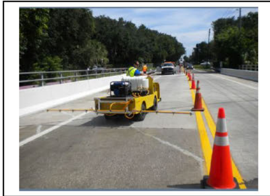
Figures 2 and 3: Half-cell corrosion potential testing (left) and treating bridge deck with SCP (right)
